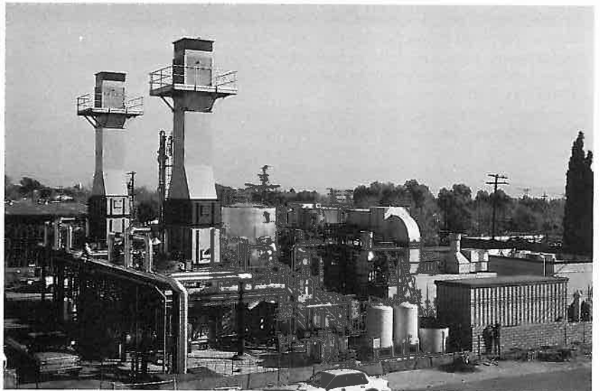
1. Cheng-cycle cogeneration system meets NO x emissions limits at citrus processor; it injects steam into a gas turbine, reducing operating temperatures
